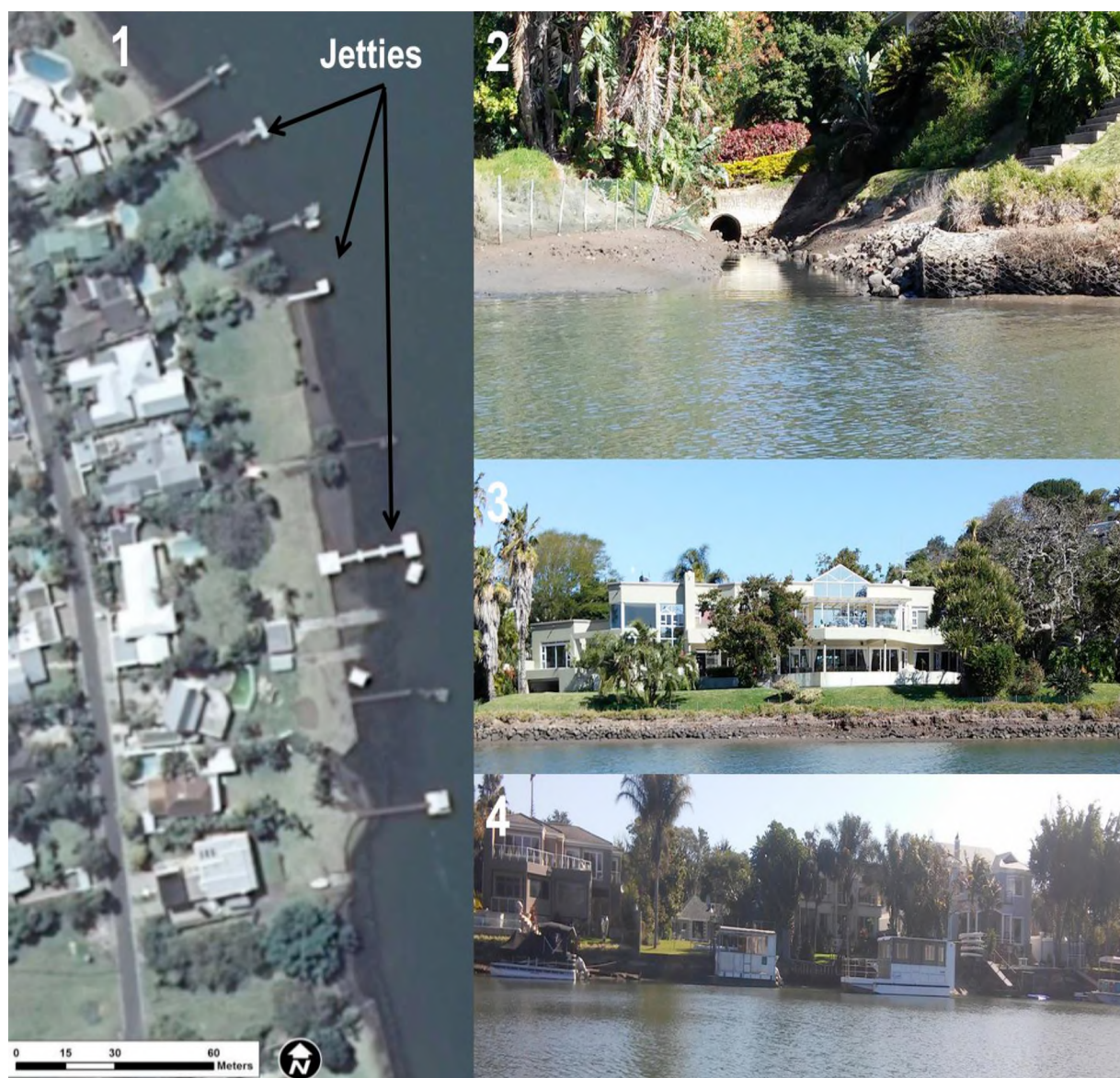
Figure B6: Modification along the lower reaches of the Nahoon Estuary. 1: Jetties along the bank; 2: One of the stormwater drains along the estuary; 3: Example of the town house occupying the river banks with artificial bank stabilisation; 4: Recreation boats floating throughout the estuary (Use is high during peak holiday times) (Images: MEGA 2013, Cotiyane 2014, 2015).
