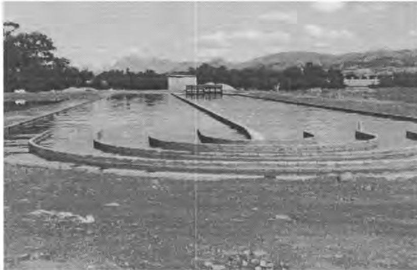
Figure 7.4.1. The 2 500 m 2 high rate algal pond at Mossop Western Leathers, Wellington.
