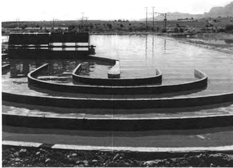
Figure 7.4.2. Flow regulating walls of the 2 500 m 2 high rate algal pond at Mossop Western Leathers, Wellington.
