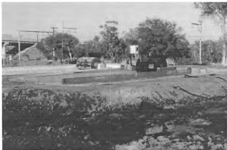
Figure 5.3.1. Photograph of the two 80 m 2 pilot high rate algal ponds at Mossop Western Leathers, Wellington.
