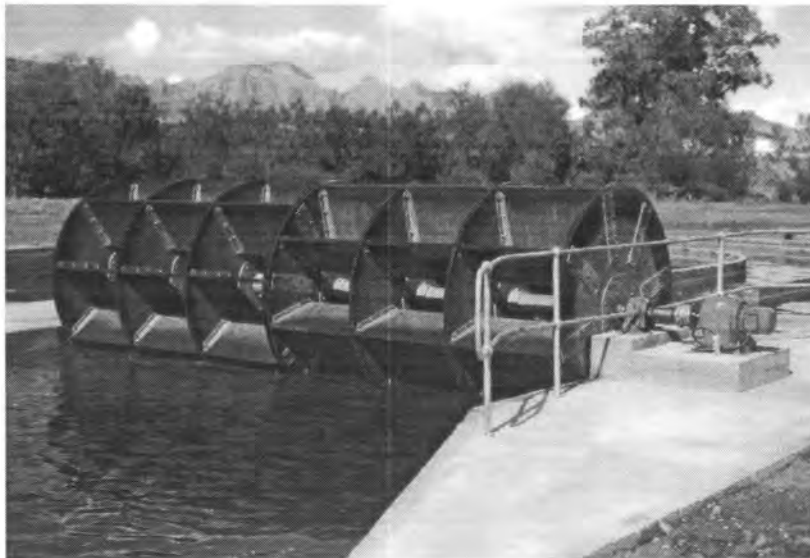
Figure 7.4.3. Paddle wheel of the 2 500 m 2 high rate algal pond at Mossop Western Leathers, Wellington.
