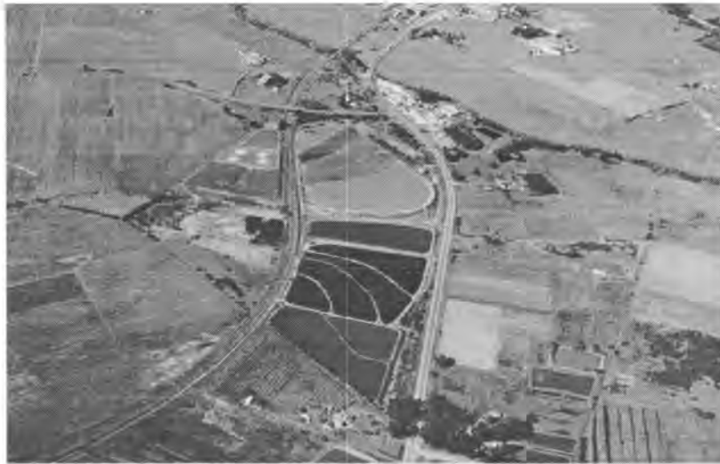
Figure 5.4.7. Aerial photograph of the WSP at Mossop Western Leathers, Wellington, showing the pronounced colour difference between anaerobic (red) and aerobic (green) ponds, and also the early effects of establishing a microalgal capping of the anaerobic ponds by recirculation.
