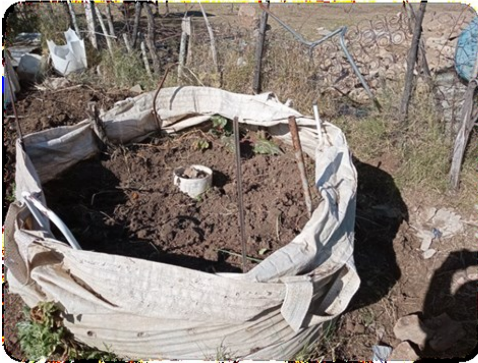
Figure7.2: Tower garden porous core construction (RU Hub Team)
