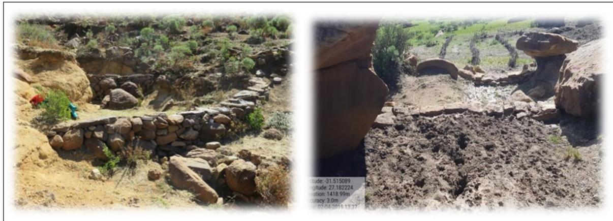
Figure 6.4: Stone pack erosion structures in the rangelands (Ru Hub Team)
