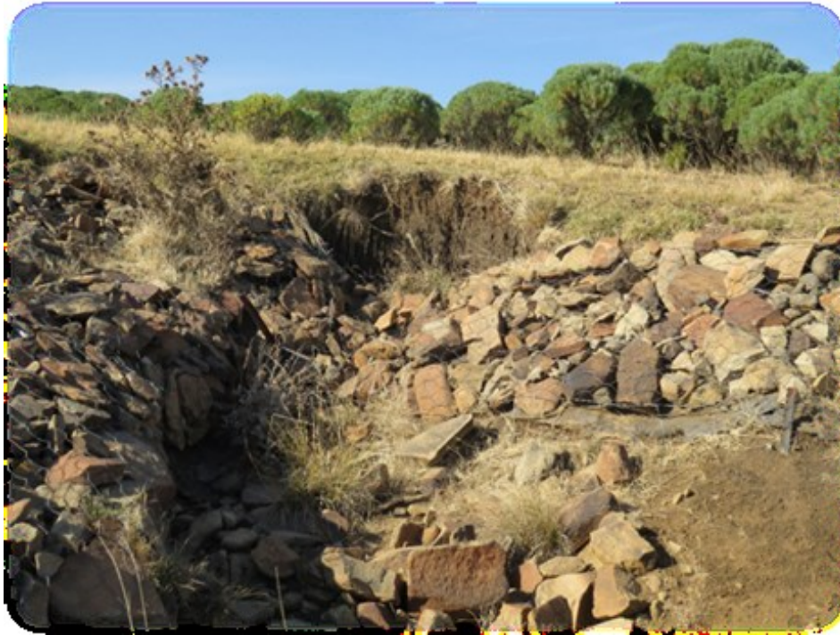
Figure 6.10: Stone pack sediment trapping structures (RU Hub Team)
