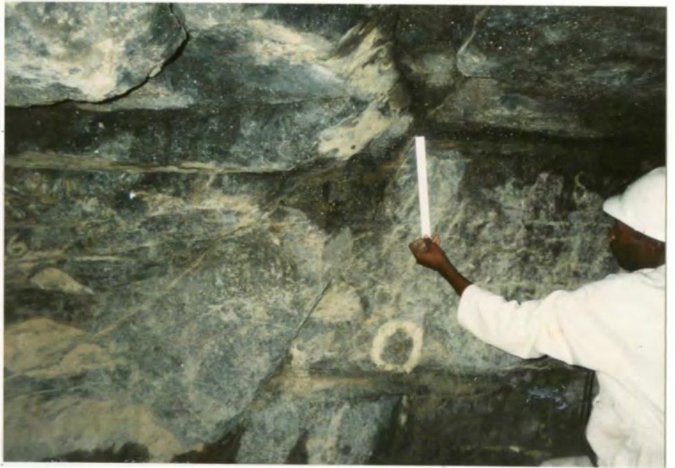
Fig 3.14 Unki stope. Step fault in 2 level north-raise (looking south).
