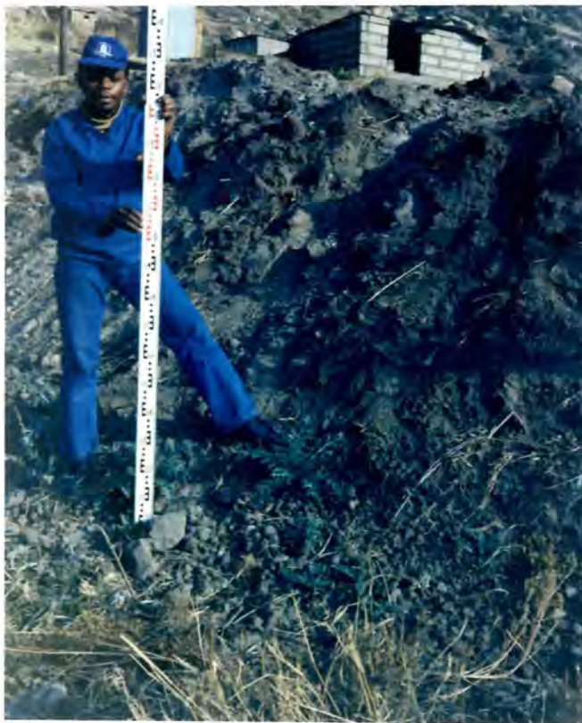
Plate 19 Gully filled with loose sediment from a construction site.
