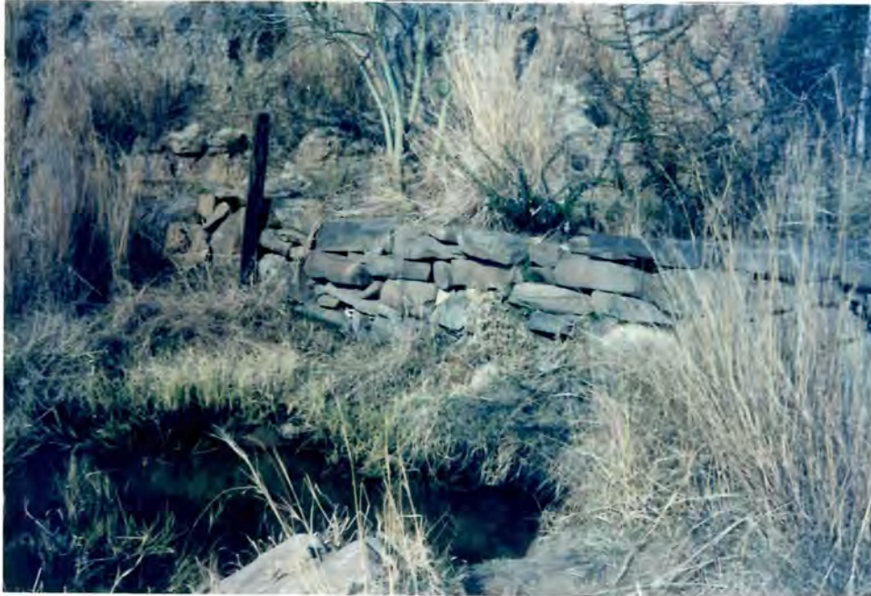
Plate 18 Check dam within gully.
