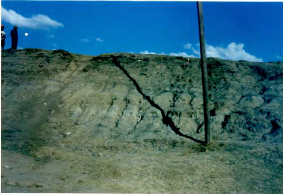
Plate 6 Parallel rills developing on a road side.
