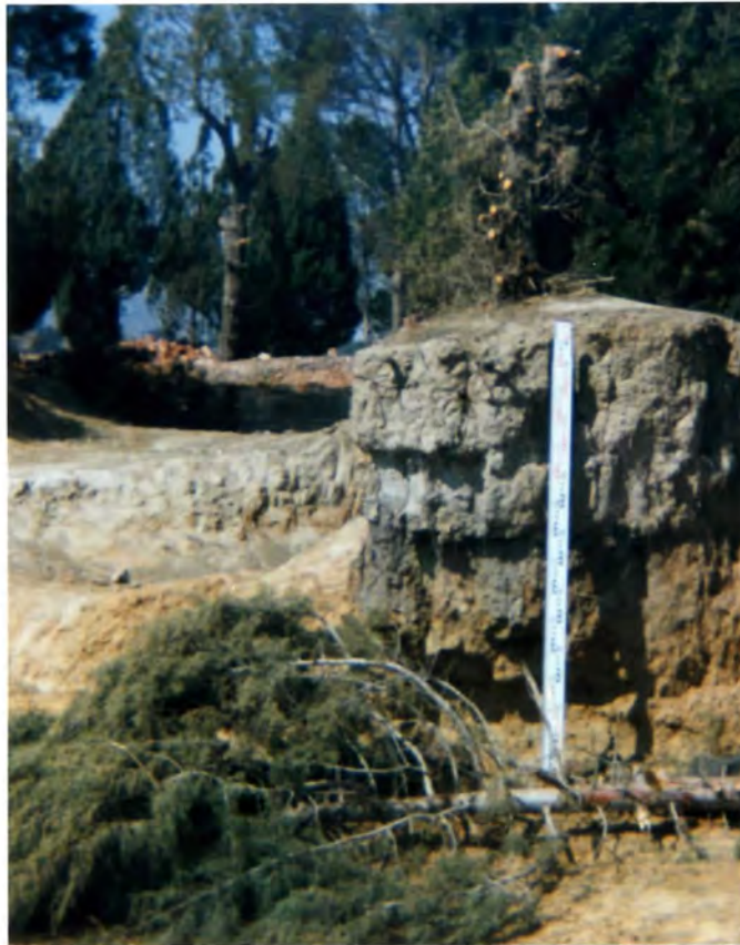
Plate 13 "Tree pedestal" on reservoir bank.
