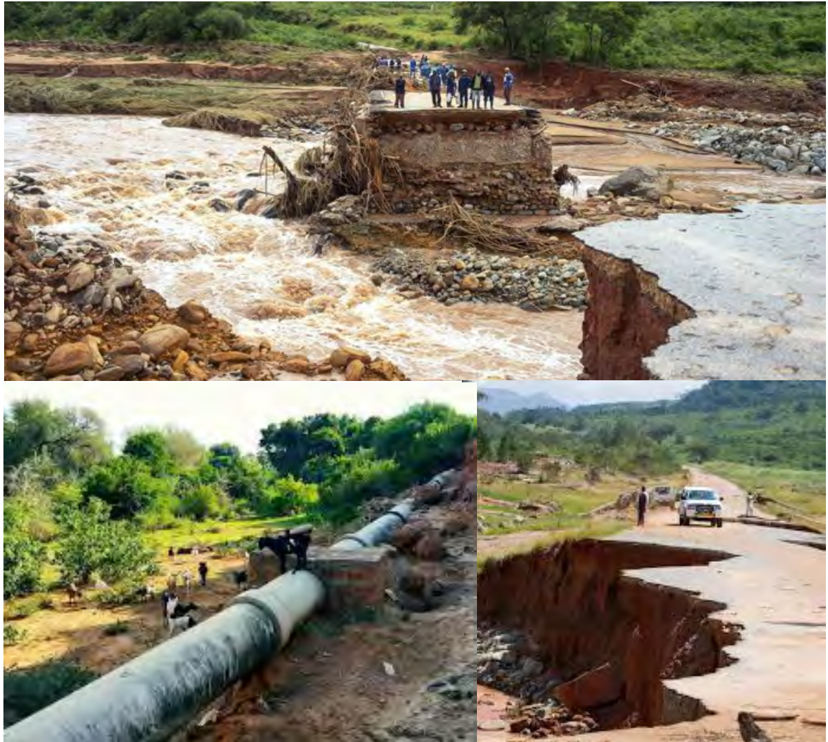
Figure 5.10: Nyanyadzi irrigation pipeline and the situation after the Cyclone Idai
