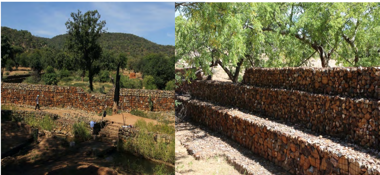
Figure 4.9: Silt trap (gabion) at the Nyanyadzi Irrigation Scheme
