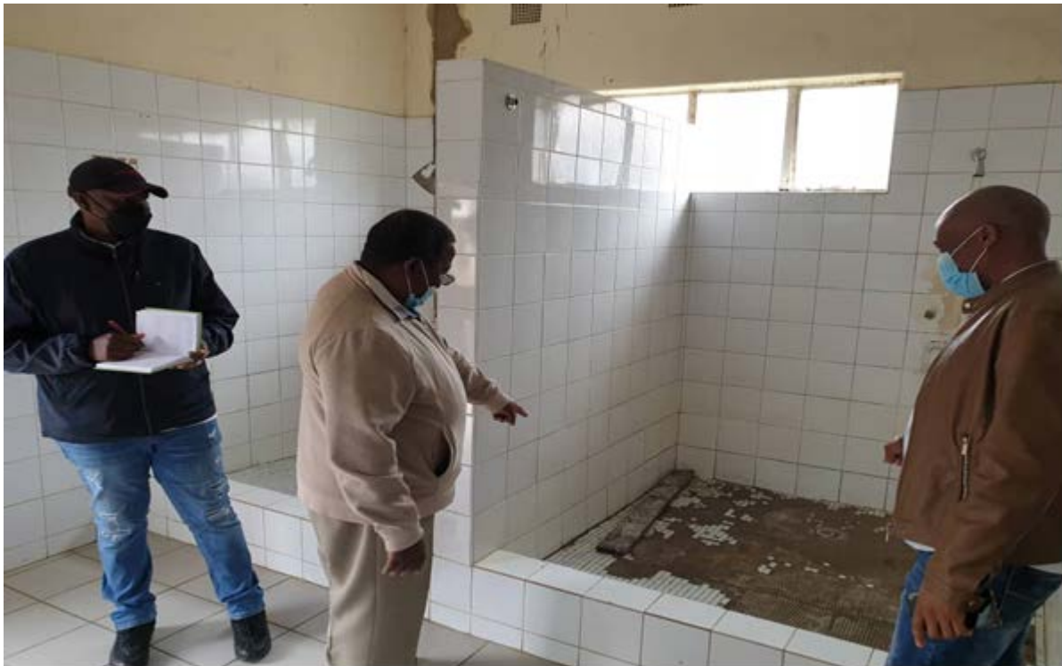
Figure 7.8: Inspection of hostel bathroom
