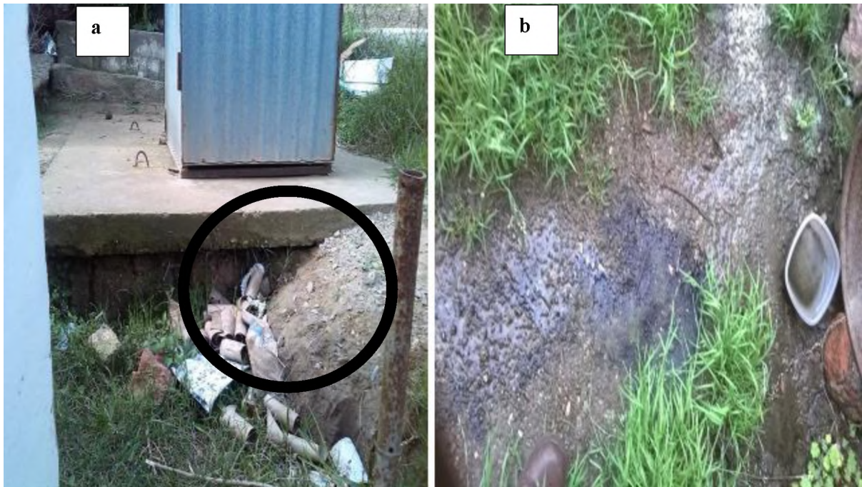
Figure 21. An image of the support concrete slab for the superstructure of the pit latrine showing an area where the sludge leaches during rainy days or seasons. b. the leaching of the faecal sludge from the pit latrine
