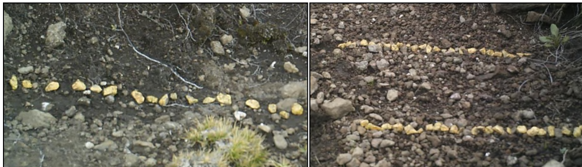
Figure 2.2. Painted stone lines as reference for deformation.
