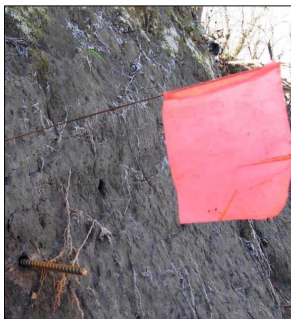
Figure 2.4. Erosion pin installed in a river bank (Alamakee County, 2015)
