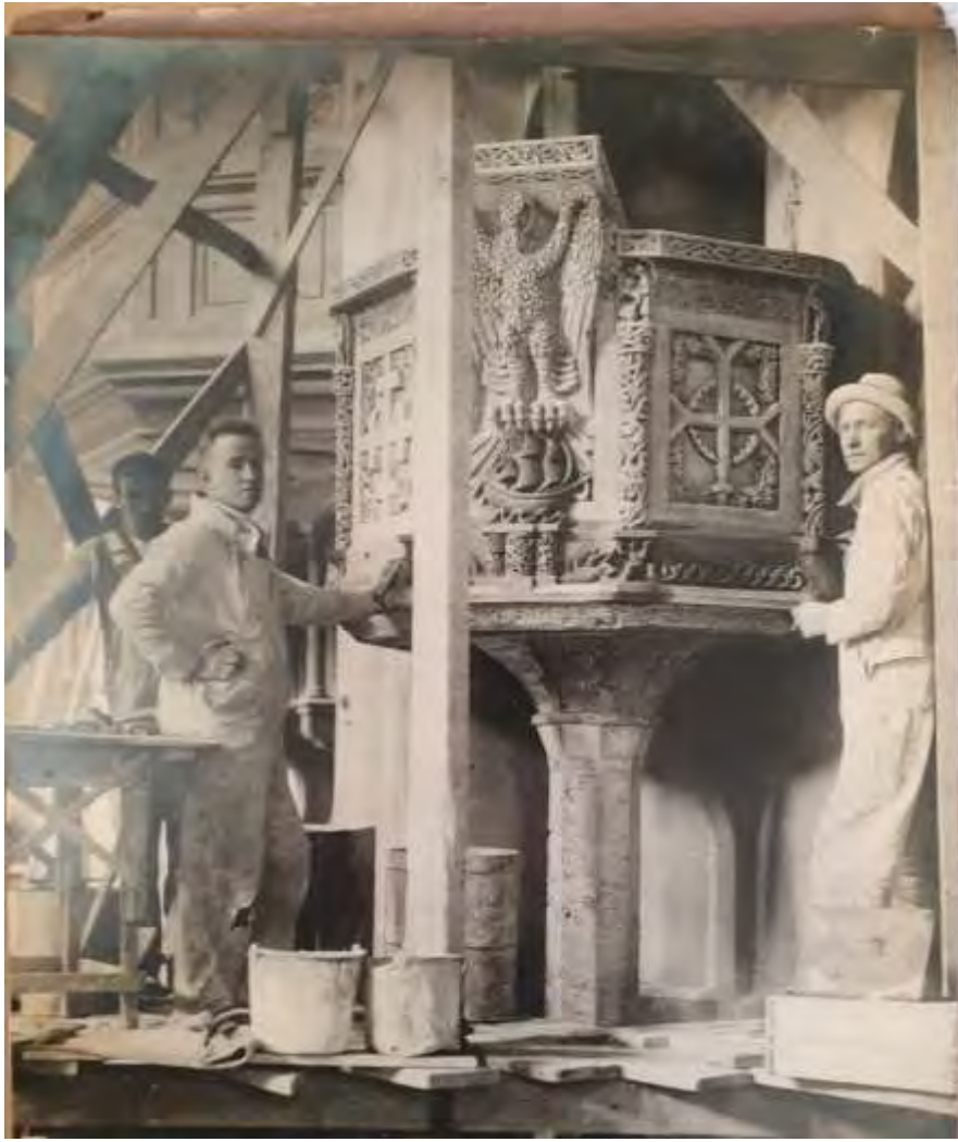
Fig. 2.5. Ned Paterson carved the pulpit in the Johannesburg Cathedral in wet cement in 1928. Courtesy of Mary Ball Paterson.
