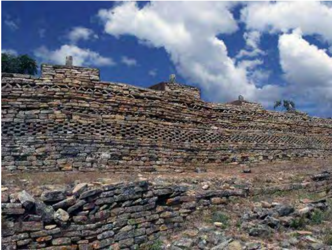
Fig. 2.2. Naletale Ruins in the Central Region of Zimbabwe is an example of a drystone capital of a complex Iron Age Zimbabwe state. What is unique and impressive about the wall at Naletale is that it carries the most dominant elaborate patterns associated with drystone wall constructions i.e., chevron, single and double chequers, dentelle, and herringbone. Source: World Monuments Fund.
