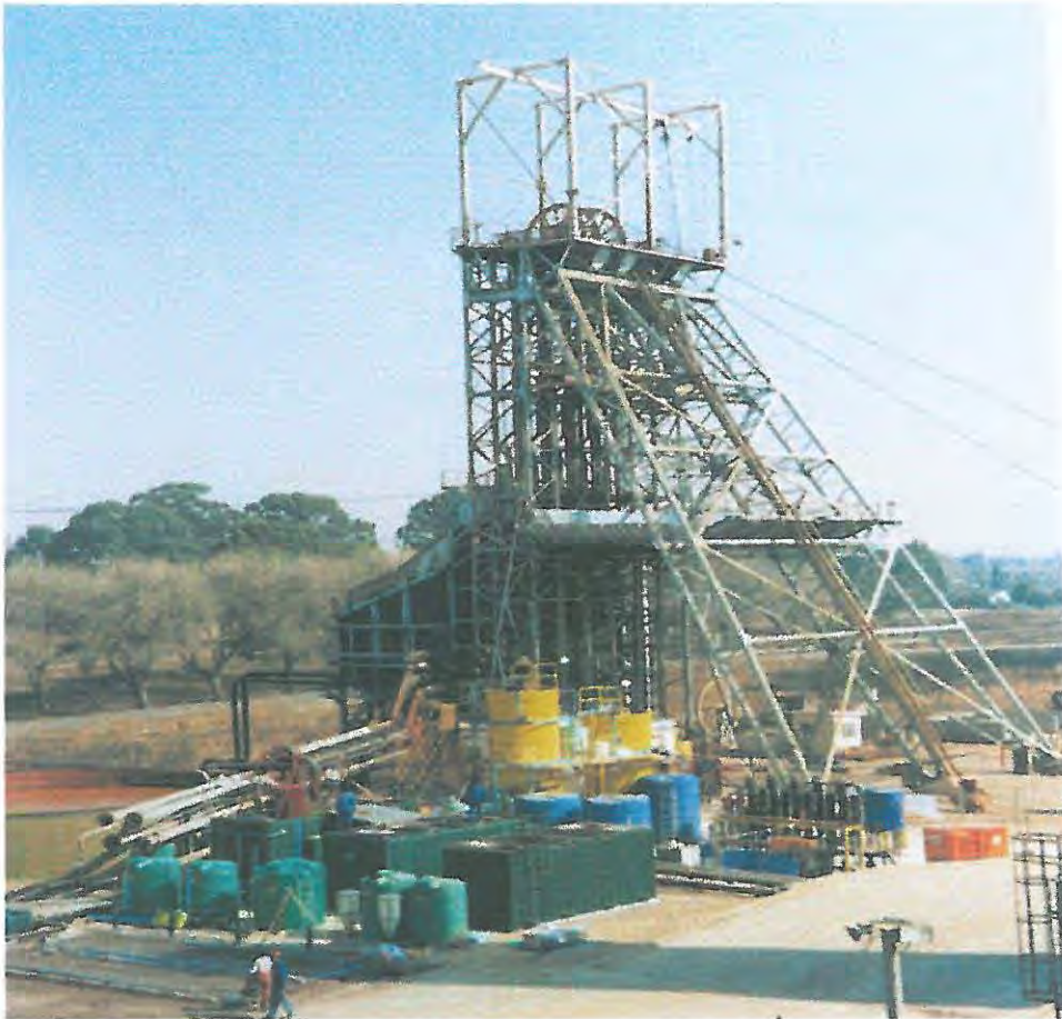
Figure 2.4 Headgear at the No.3 shaft Grootvlei Mine with the Rhodes BioSURE Process pilot plant assembled in the foreground.
