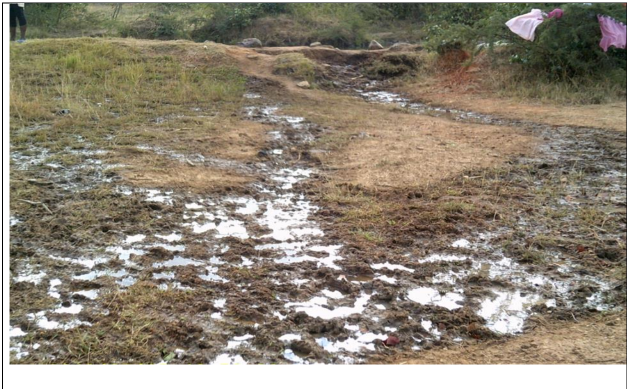
Figure 4: Seepage from Main Canal
