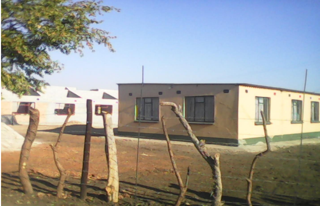
Figure 14: Land-seeker's Homestead under Construction on an Infill
