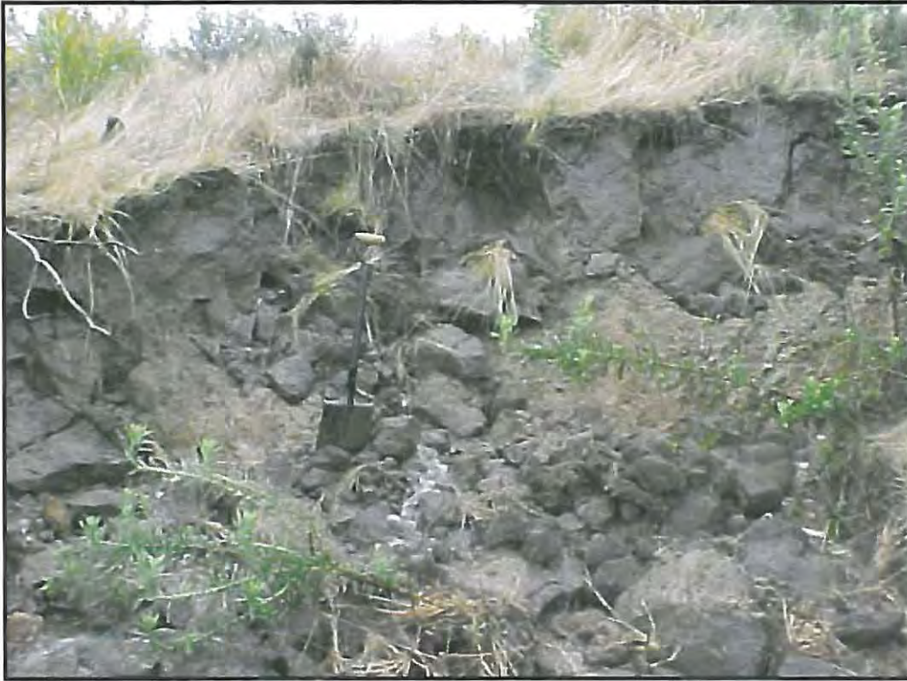
Plate 5.2: Soil slumping on the catchment slopes
