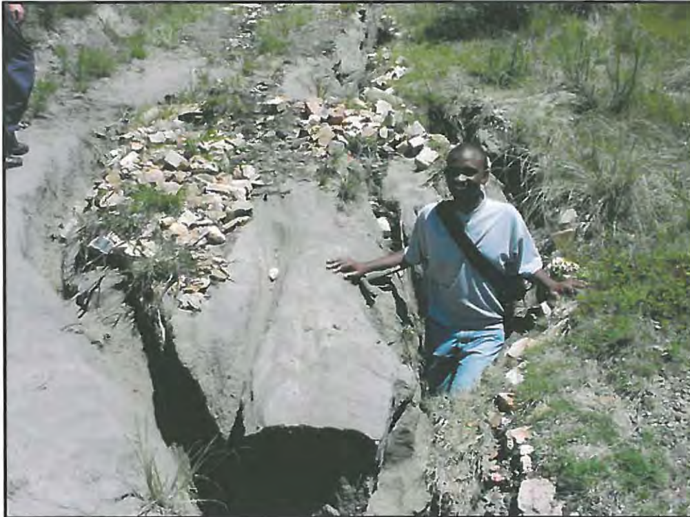
Plate 5.1: The extent of erosion on the road by-passing the wetland site (Courtesy of Kate Rowntree)
