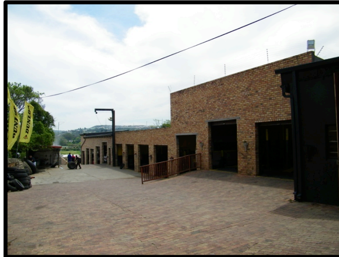
Figure 3.2 Warrick's yard seen from the frontstage/reception area
