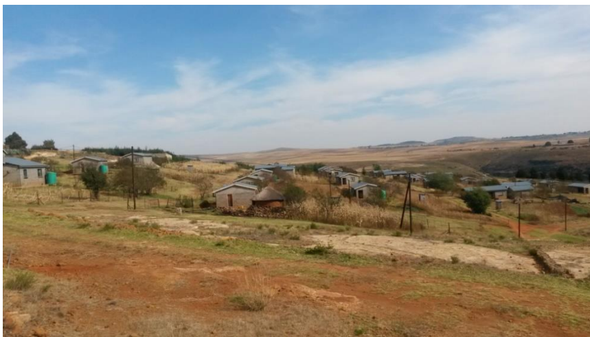
Figure 9.1 A village designed for Phase 1B resettled people at Ha-Ratau, Maseru, Lesotho
