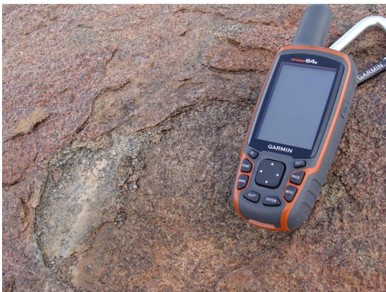
Figure 7.3.5: Spalling crusts on Northern Buttress, Vesleskarvet
