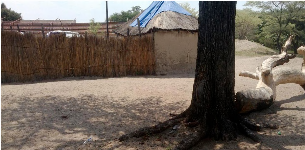
Figure 4.5: Walls of the house built with mud and roof thatched with grass
