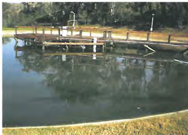
Figure 2-1: The PFP component of the IAPS pilot plant, with a fermentation pit underneath
