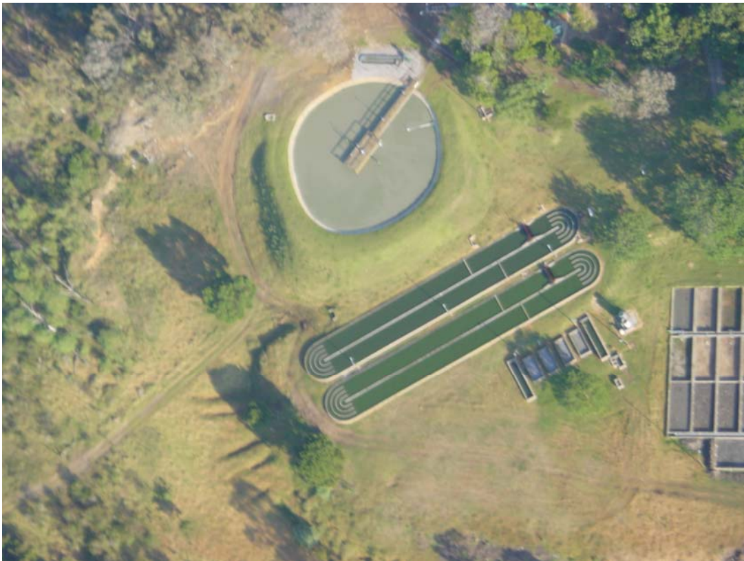
Figure 2.1: The integrated algal ponding system plant at the Experimental Field Station, showing the primary facultative pond (top) and high rate algal ponds, algal settling ponds and drying beds below.
