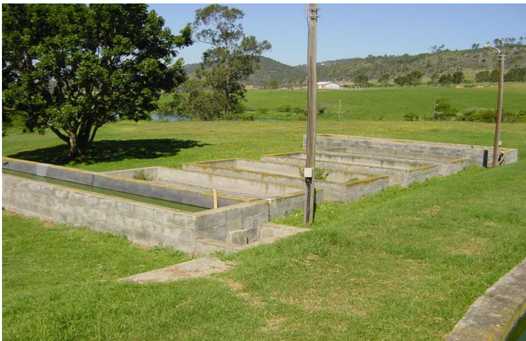
Figure 2.5: The four algal drying beds between the two algal settling ponds.
