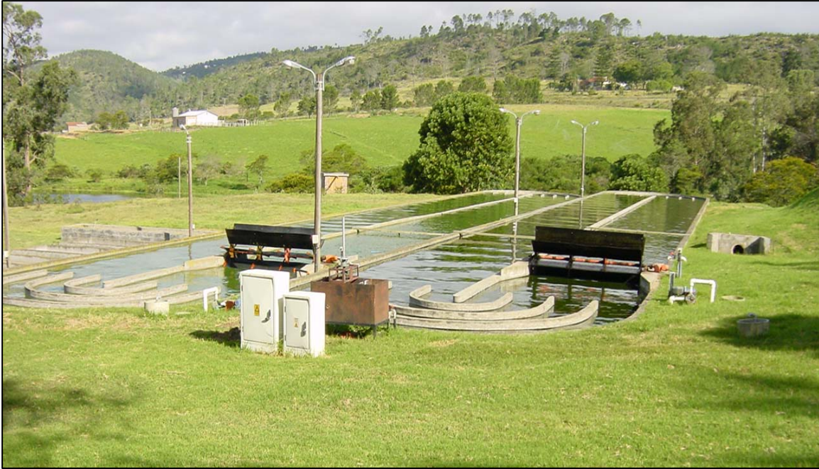
Figure 2.3: High rate algal ponds, depicting channel dividers.
