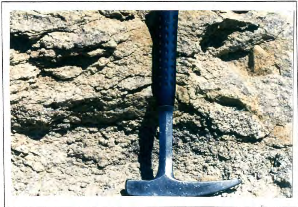
Plate 2.4 Highly fractured yellow rock typical of quartz-sericite-pyrite alteration of the Marinkas Kwela Granite.
