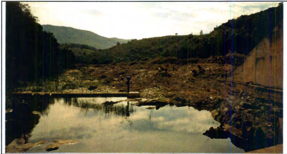
Plate 5: Above weir 1 looking down river after felling of trees.
