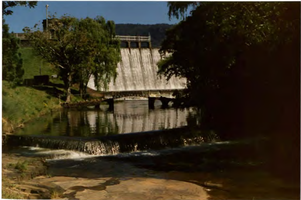
FIGURE 2.1 Maden Dam in summer when the dam is overflowing.
