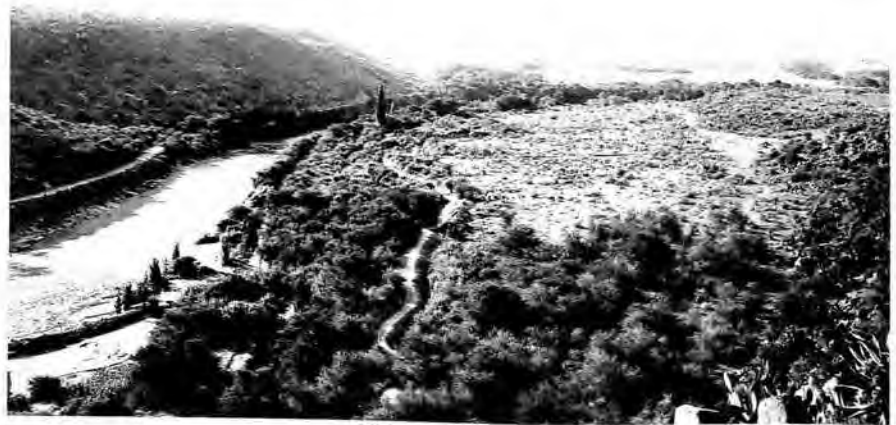
Plate 1 : View of the proposed site of the Van Rynevelds Pass Dam wall on the Sundays River.
