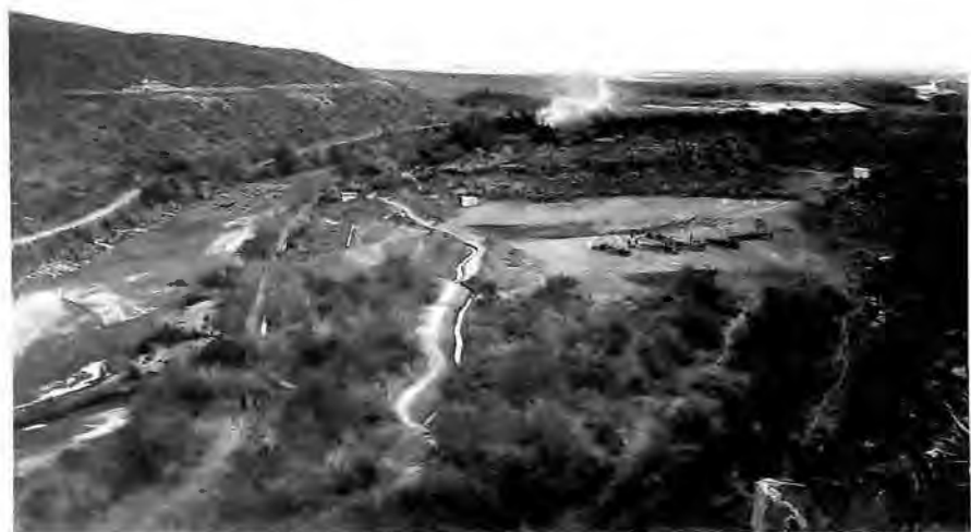
Plate 2 : Construction on the Van Rynevelds Pass Dam wall, and earth-lined canal from the "Mackies Pits" - July 1921.
