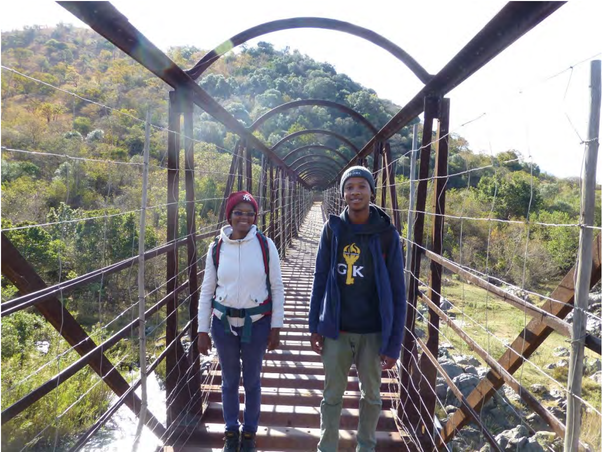
A bridge across the Komati river in the Songimvelo Nature Reserve. In the background of the photo are the mountains of the Kromberg type-section.
